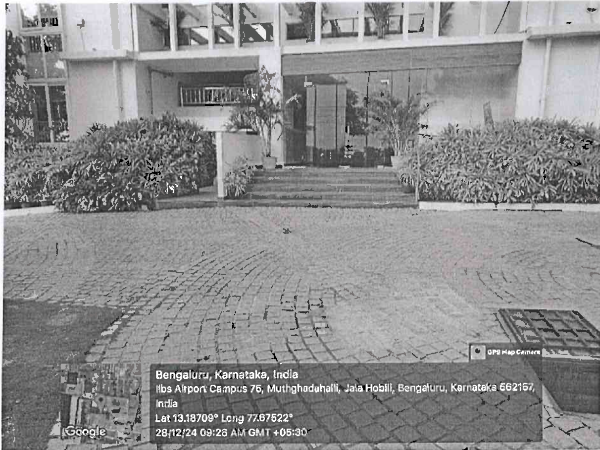
Floor modified for better Water Seepage
